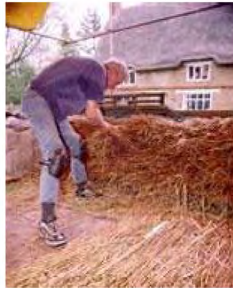
Figure 7 Drawing threshed 'long straw' straw from a bed (Northants)
